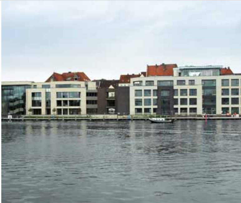
New water front at the inner harbour of Emden, Lower Saxony
