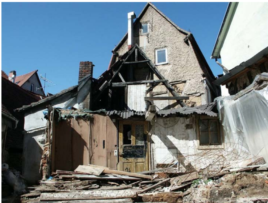
Figure 11: Demolition of a timber frame building in Partenstein, Spessart, Germany
